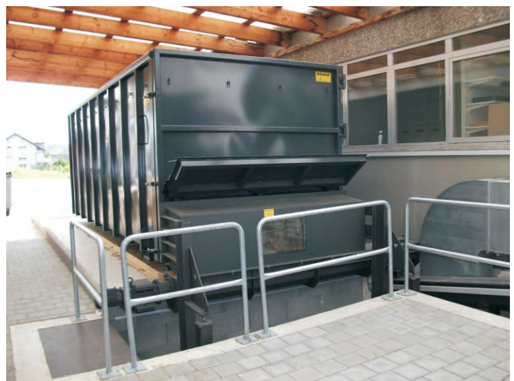
Pushing floor change container for wood chips: The container is picked up, filled and returned to the Nolting docking station on the premises by the local chips supplier.
