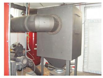
The de-duster (heat insulated) includes an induced draught and an easily changeable ash bin.
