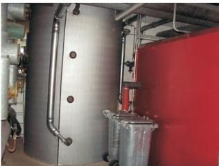
Buffer storage tank including insulation Water filling volume: 5000 liter
